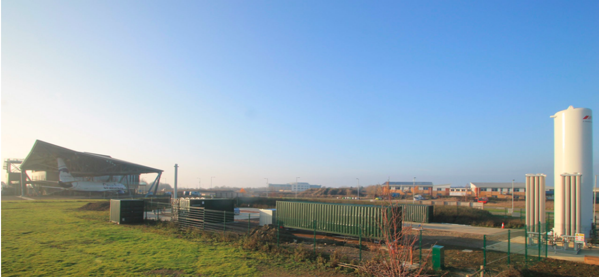
Fig. 24 Construction of hydrogen production facility [44]
