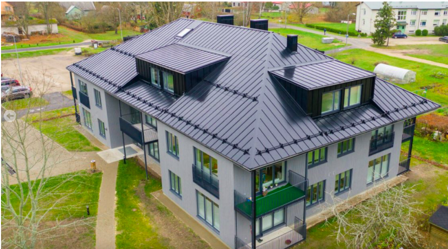
Fig. 22 PV roof example from Roofit Solar company - Haapsalu rental house [38]
